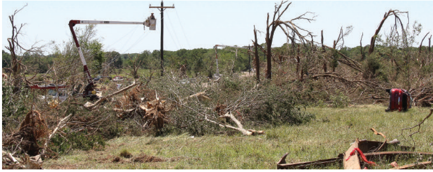
The April 29 tornado damage in Trinity Valley EC's service territory near Canton
